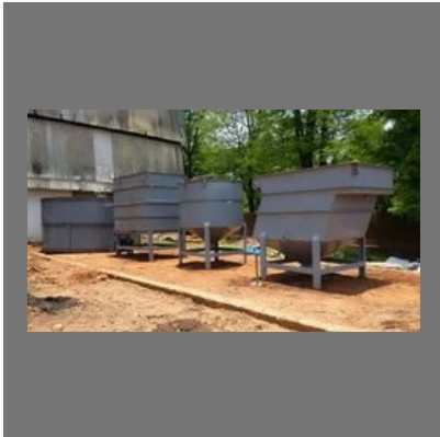
Compact Effluent Treatment Plant
