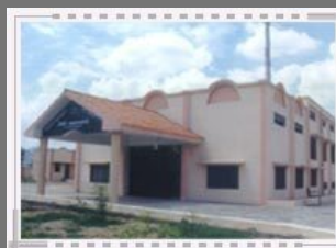
Completed Project Building
