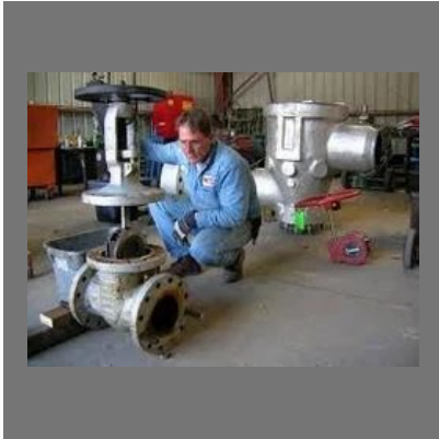
Onsite Gate Valves Repairing
