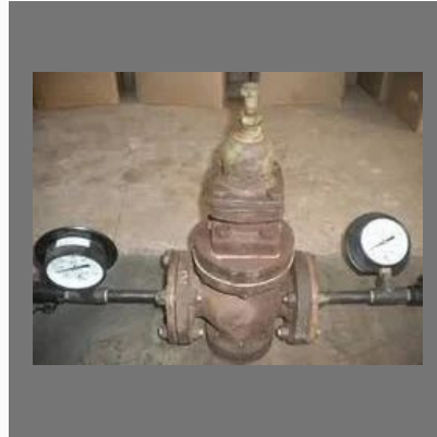
Pressure Reducing Valve Repairing
