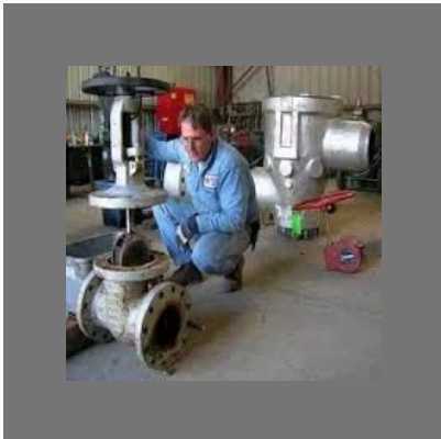
Sluice Valves Repair
