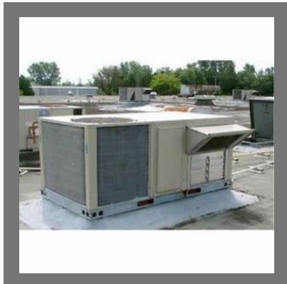
Rooftop Air Conditioner
