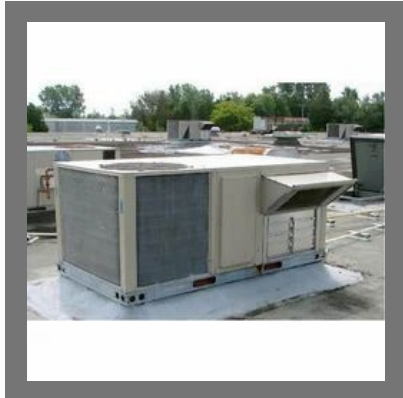
Rooftop Air Conditioner
