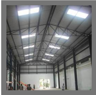
Metal Roof Trusses
