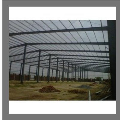
PEB Structural Shed
