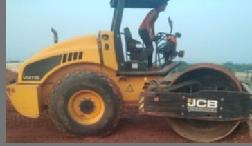
Road Construction Service
