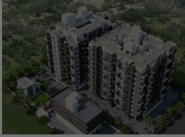
Commercial Building Construction Service
