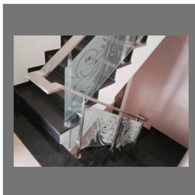
Stainless Steel Stair Railing
