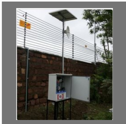
Solar Fencing Installation service
