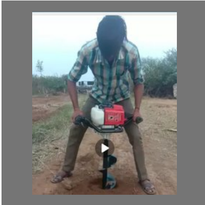
Earth Digging Services
