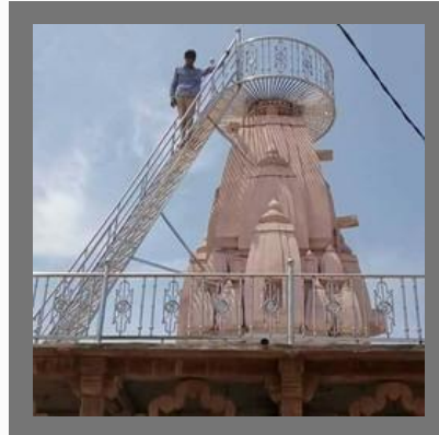
SS Mandir Railing
