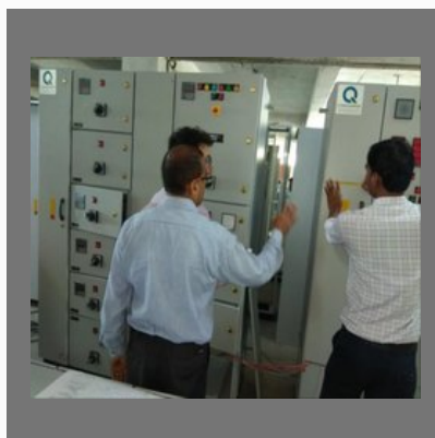
Electrical Design Service
