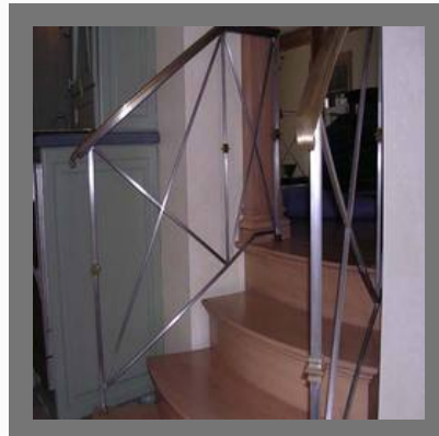
SS Hand Railing
