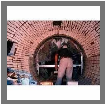
Refractory Brick Lining Service
