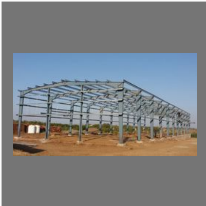
Heavy Structural Erection Service
