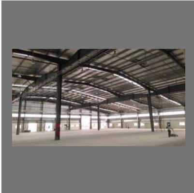
Pre Engineering Building Shed with Jack Beam
