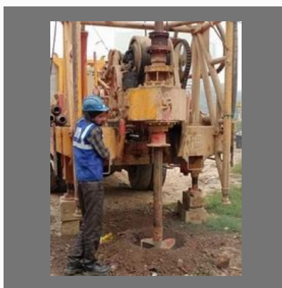
Boring Work in Delhi
