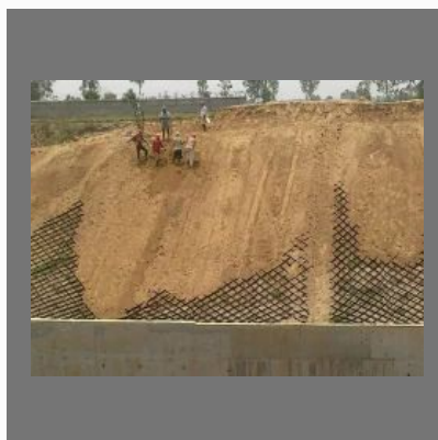
Slope Stabilization Work
