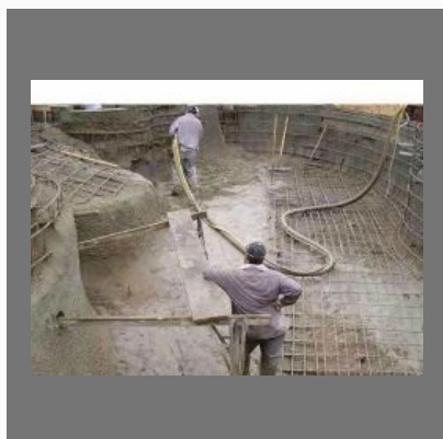
Guniting Shotcreting Drilling Work
