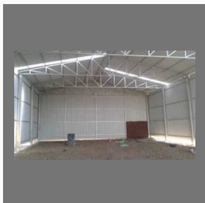
Industrial Roofing Shade
