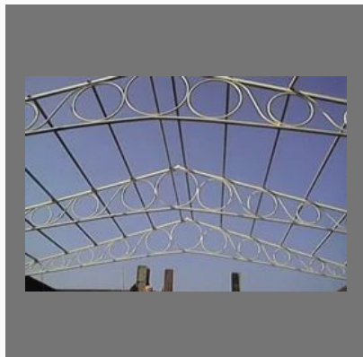
Industrial Roofing Structure
