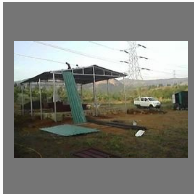
Sheet Roofing Structure Shade
