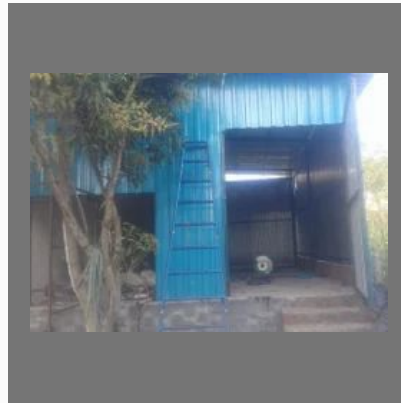
Industrial Sheet Roofing Shade
