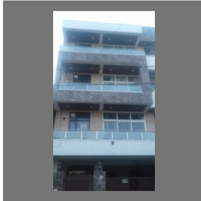
SS Balcony Railing
