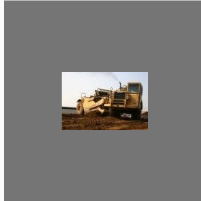
Concrete Road Construction
