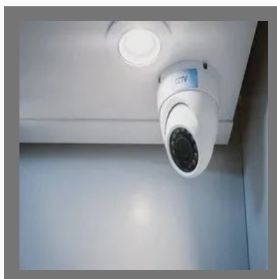
Wireless Cctv Camera Installation Services
