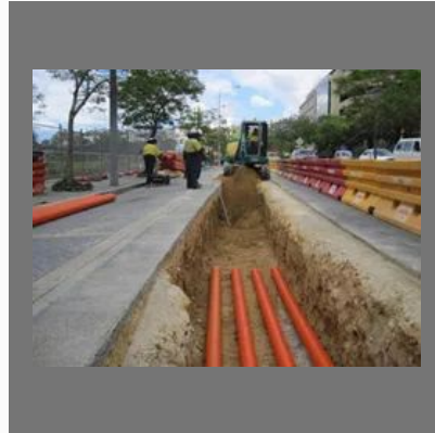
Underground Laying Optical Fiber Cable Services
