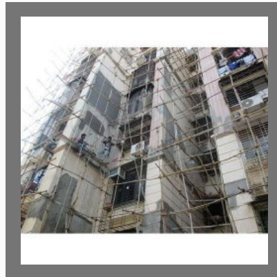
Hospital Renovation Services
