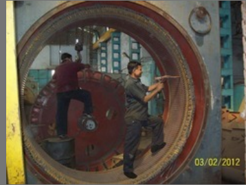
HT Alternator Winding Repairing Services
