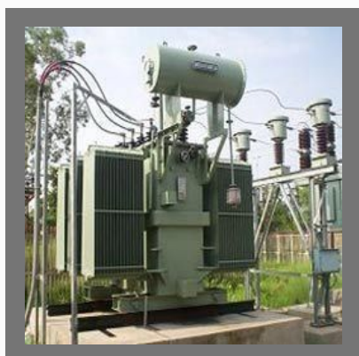
Transformer Maintenance Services
