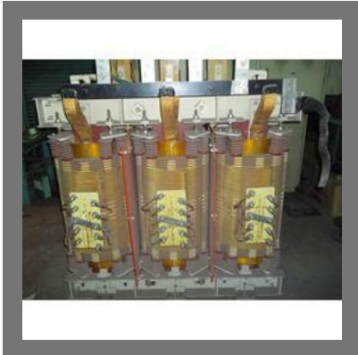
Transformer Repairing Services
