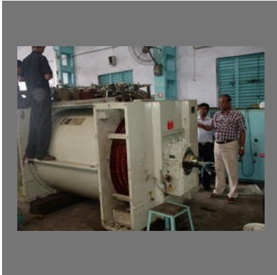
Generator Repairing Services
