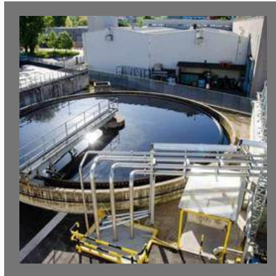
Sewage Water Treatment Plant
