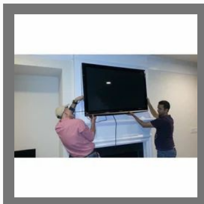
LCD TV Installation Service
