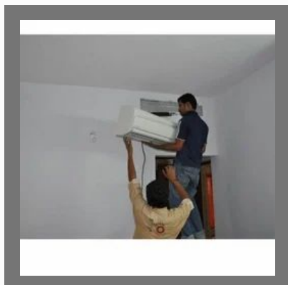
AC Installation Services
