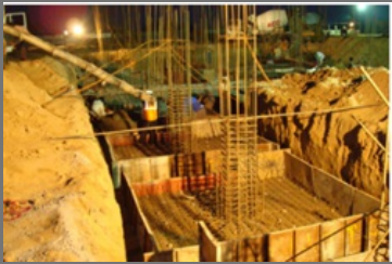
Factory Building Construction Service
