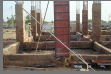
Shopping Mall Construction Service
