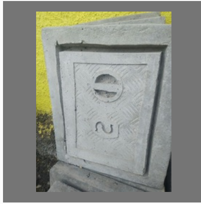
Concrete Manhole Cover
