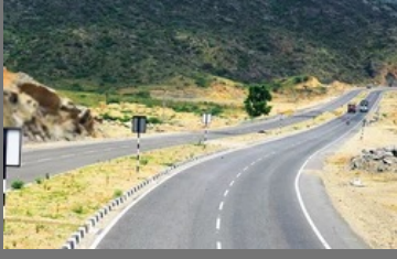
Road Construction Service
