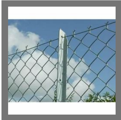
Chain Link Fencing
