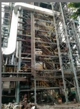
Boiler Erection Service
