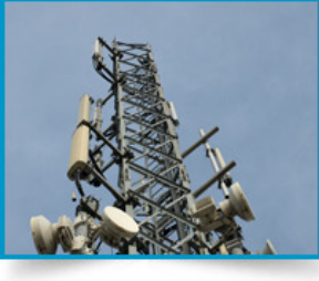
Commissioning and Integration Cabling.
