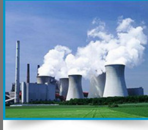
Service Contracts Of Power Plants Inclusive Of Pm & Apm.
