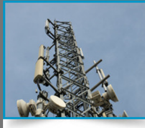
Installation and Commissioning of add carriers.
