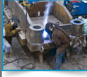
Pneumatic Pipe Lines Fabrication for Industrial Purposes
