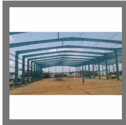
Pre Engineered Building Structure
