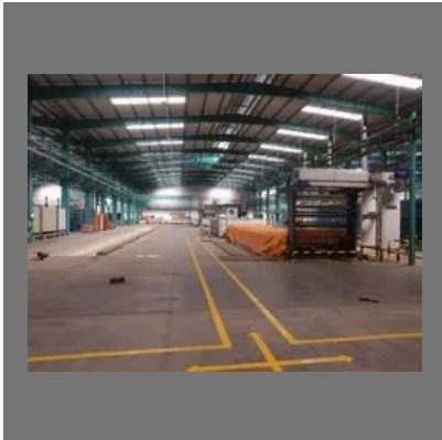
Project Management Consultancy
