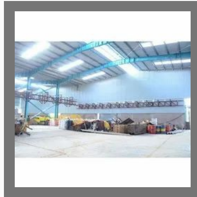
Steel Pre Engineered Building
