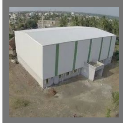
Commercial Buildings Construction Service
