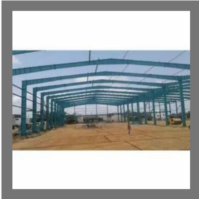
Pre Engineered Building Structure
