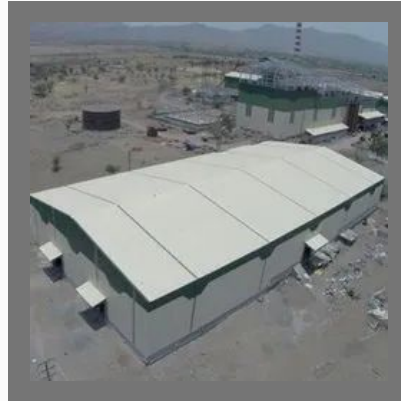
Warehouse Construction Services
