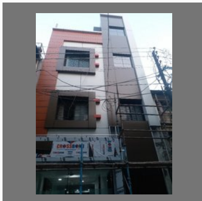
Aluminium acp work & glazing work
