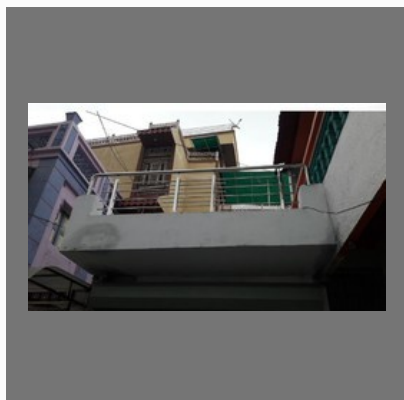
SS Balcony Railing
