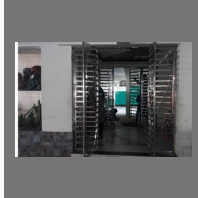
SS Grill Main Gate
