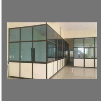
Glass Work For Portable Cabins
