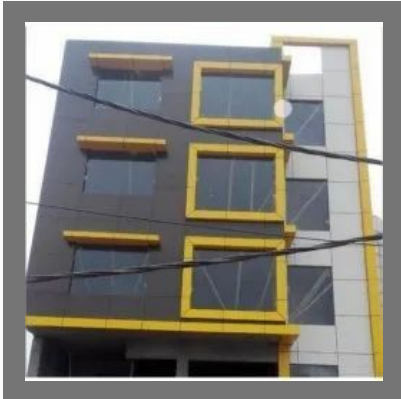
ACP Glass Glazing Work
