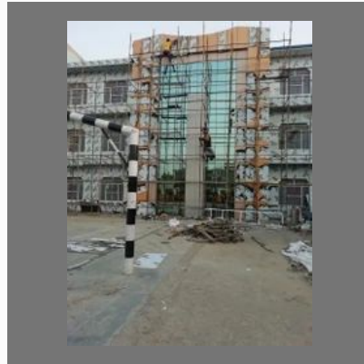
Acp Structural Glazing
