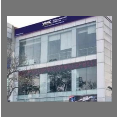
Wall Cladding Acp Sheets
