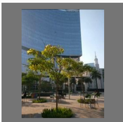
Aluminum Curtain Wall
