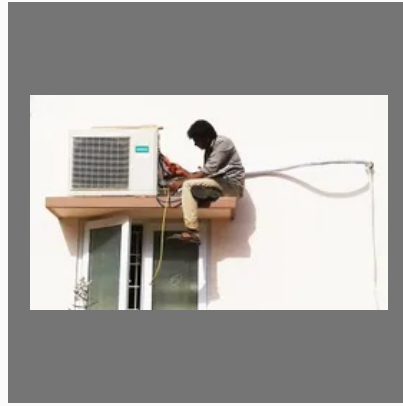
Air Conditioner Maintenance Services
