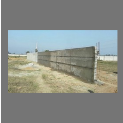
Boundary Wall Contractor
