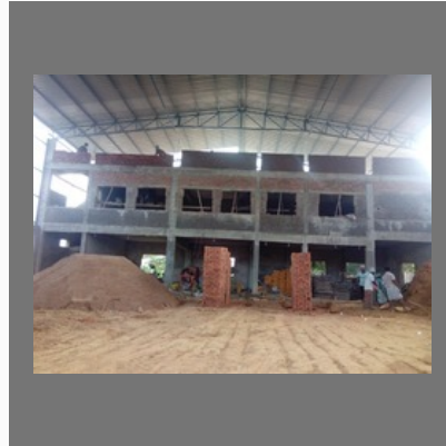
Factory Shed Contractor In Redhills
