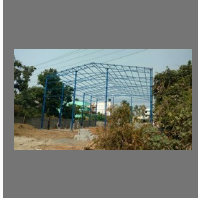
Badminton Court Construction Services
