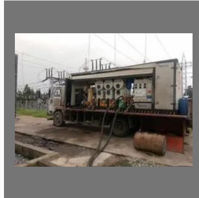
Transformer Oil Filtration Services
