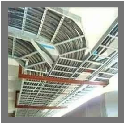
HT LT Cable Laying
