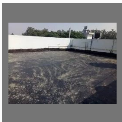
Roof Waterproofing Services
