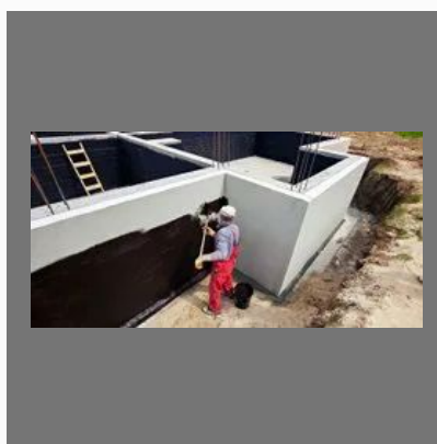
Foundation & Basement Waterproofing Service
