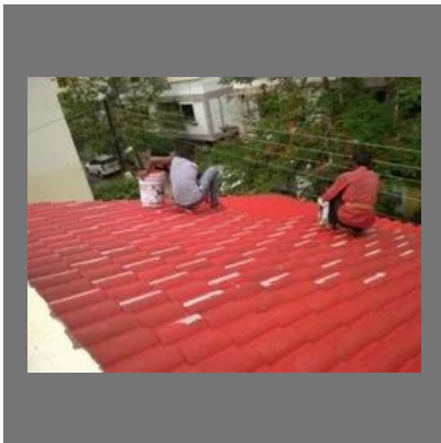
Residential Roof Waterproofing Services
