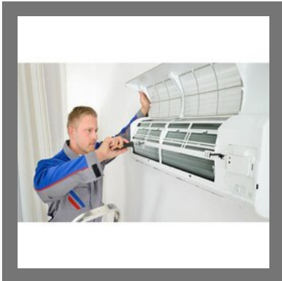
Split AC Repairing Service
