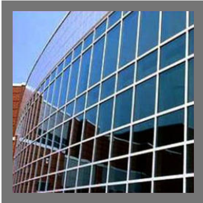
Outdoor Glass Installation Work
