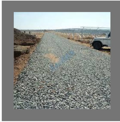
Road Construction Service
