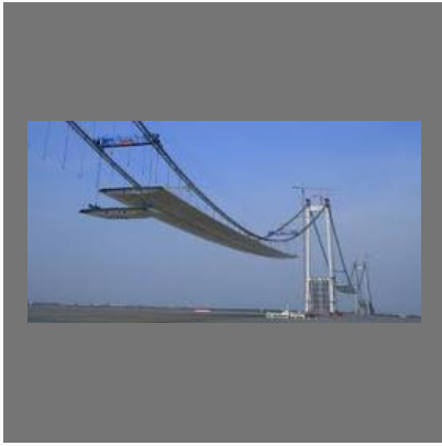
Bridge Construction Services
