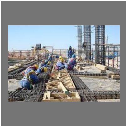
Flyover Construction Services
