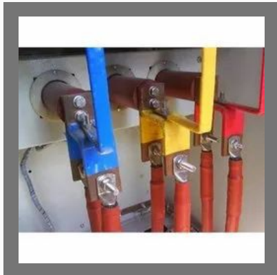
LT Cable installation & Termination Services
