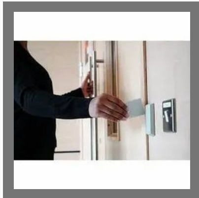
Door Access Control Service
