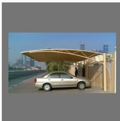
Car Parking Shed Fabrication
