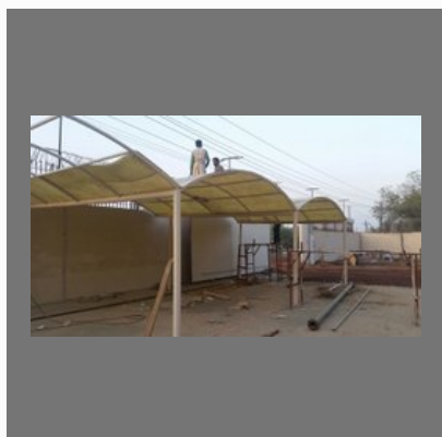
Parking Shed Fabrication
