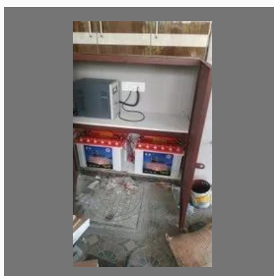
Inverter Repairing Services
