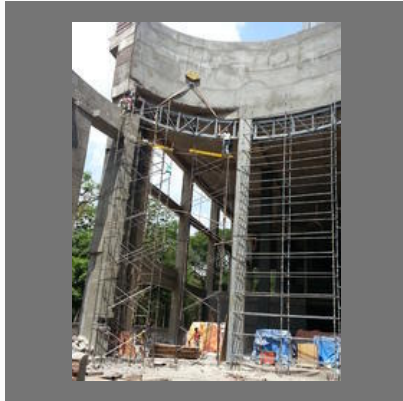
RCC Column Strengthening Service
