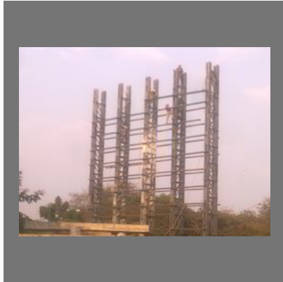
Heavy Fabrication Work
