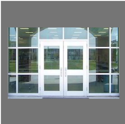
Glass Door Repairing
