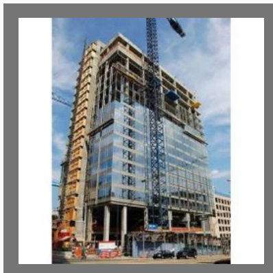
Hotel Construction Service
