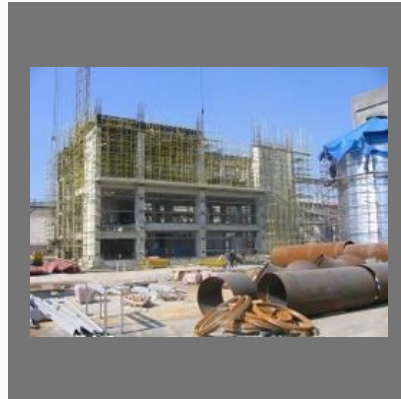
Commercial Construction Service
