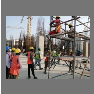
Scaffolding Inspection Services
