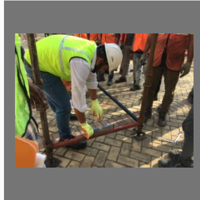
Scaffolding Inspection service
