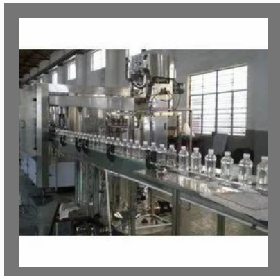
Packaged Drinking Water Plant
